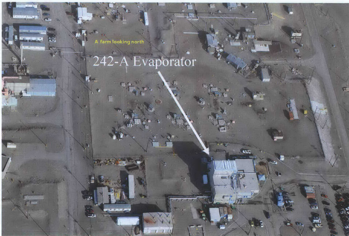
Figure 5. 242-A Evaporator Aerial View.
